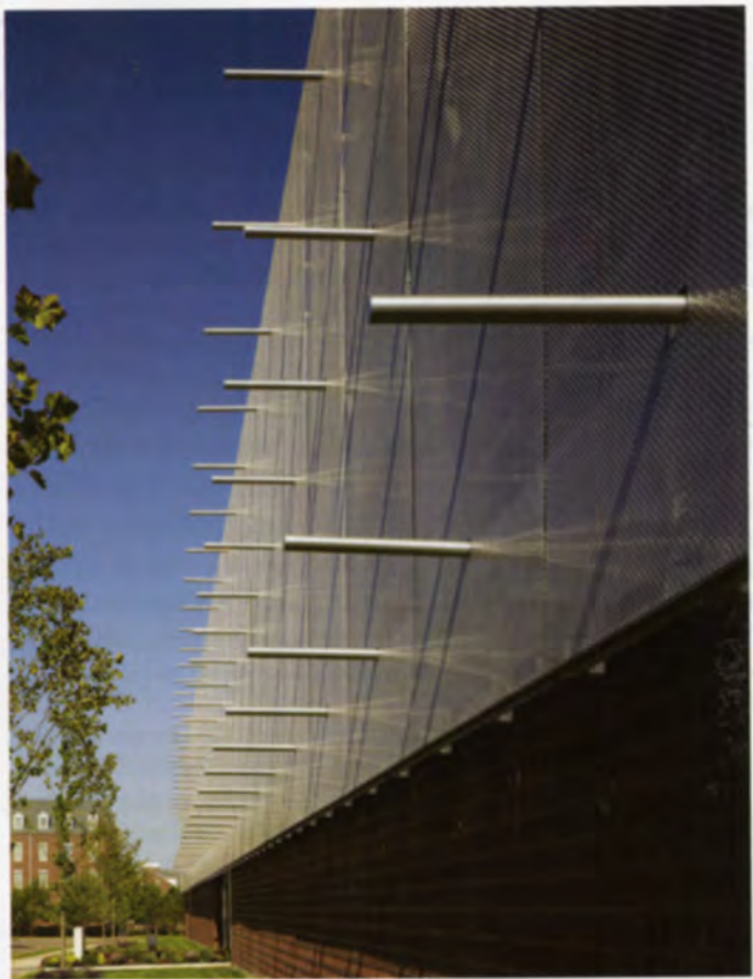
The metal screen exterior with four foot outriggers that provide linear shadows hinting at the use of the facility.
