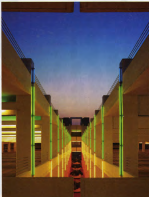
The center atrium at the Chesapeake Car Park allows sunlight to flood the interior of the garage and provides a colorful view for parkers.
