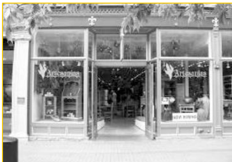
Traditional kickplates below display windows
