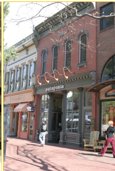
Historic Buildings, Pearl Street Mall, Boulder c. 2010 Credit: Amy Ashcraft under Creative Commons license
