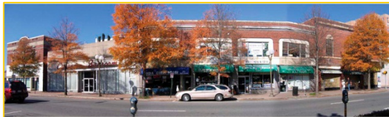
Building frontage designated for preservation Credit: Arlington County Department of Community Planning, Housing and Development, Planning Division
