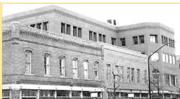
New construction set back to better integrate with older buildings
