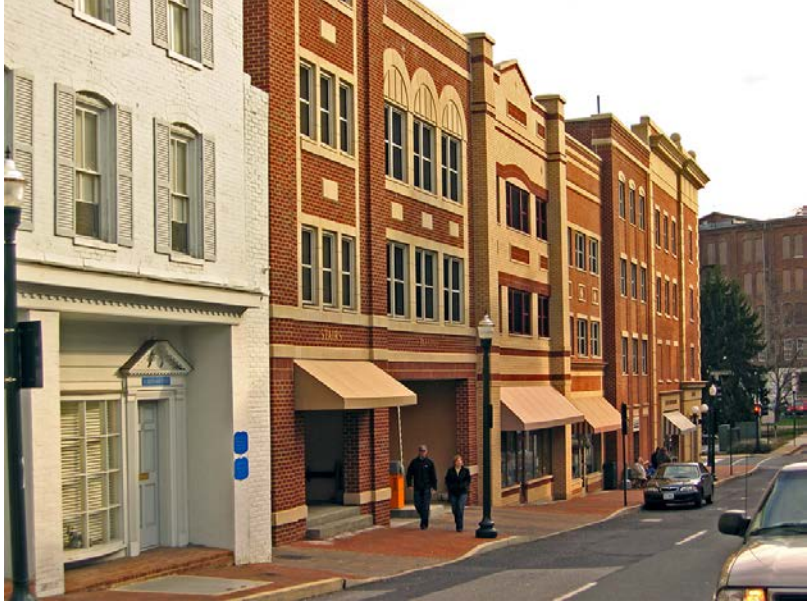
Mid-block parking structure, Staunton, VA Credit: EPA Smart Growth
