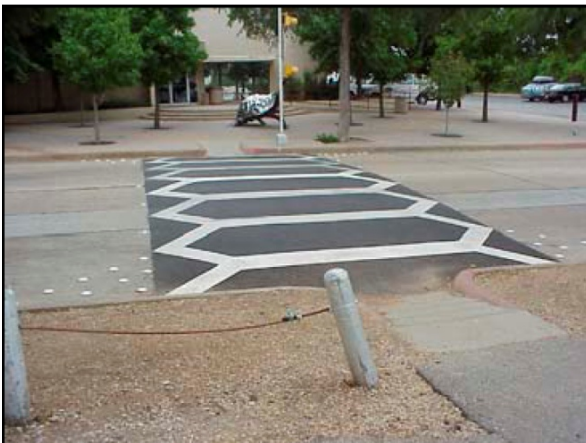
Raised crosswalk slows traffic Credit: City of Santa Barbara, CA
