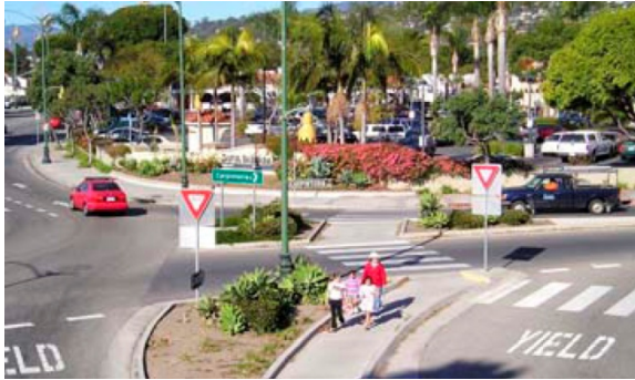
Milpas Street roundabout with wedge islands Credit: City of Santa Barbara, CA
